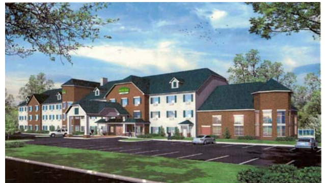
Construction has begun on the 81-room Settle Inn & Suites in Appleton, WI, which is being developed by Total Service Development, LLC as part of a multi-property franchising deal.
